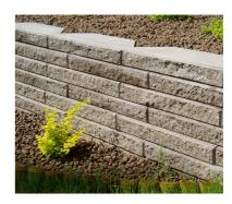
Laying should start from the cornerstone. Tighten the string marking the top of the first layer. Lay according to the string and check with a spirit level that the stones have been placed correctly. When building a wall, it is important that the first row is laid correctly.
